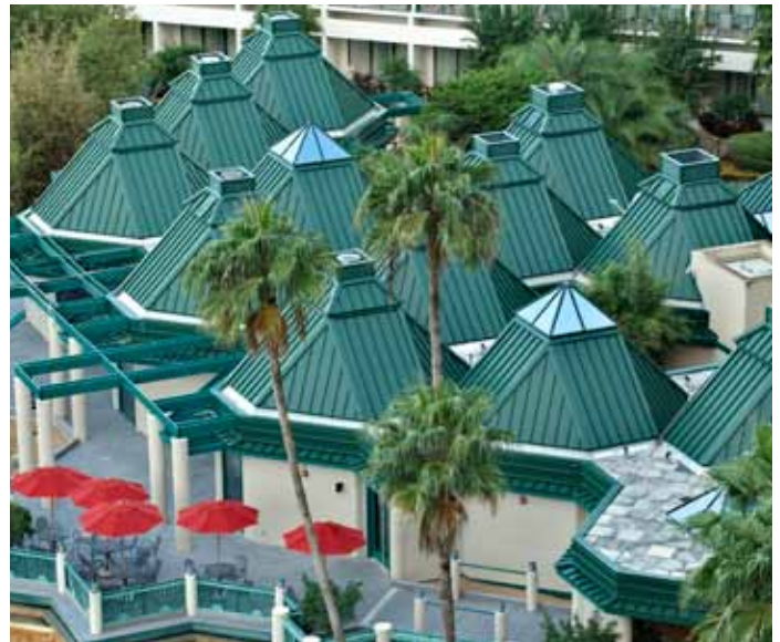
Orlando World Center Marriott - Orlando, FL Owner: Marriott Corporation Architect: Building Consultants LTD Roofing Contractor: Nations Roof of Orlando/Nations Roof of Atlanta Roofing Distributor: CRS/Commercial Roofing Specialties Color: Forest Green Profile: Snap-Clad Panels
