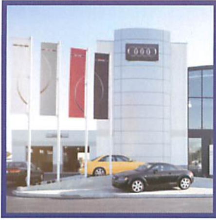
Omega-Lite panels are fabricated on-site for fast and inexpensive installation.
