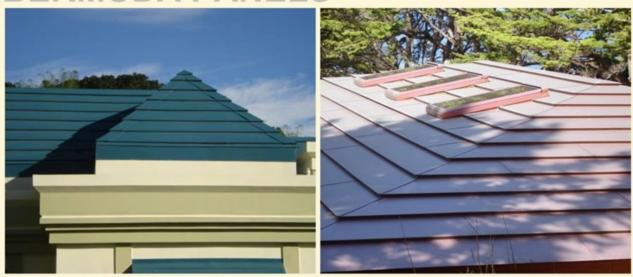
Bermuda panels have a unique internal drainage component designed to remove moisture that migrates into the system. The joints allow for controlled expansion and contraction in every direction.
