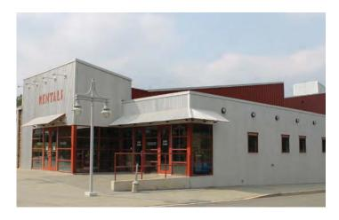
The Corrugated Panel is a traditional, economical wall or roof panel. It is installed horizontally or vertically with exposed fasteners. The panel is available in smooth or stucco embossed texture, depending on material. Ideal applications are walls, mansards and equipment screens.
